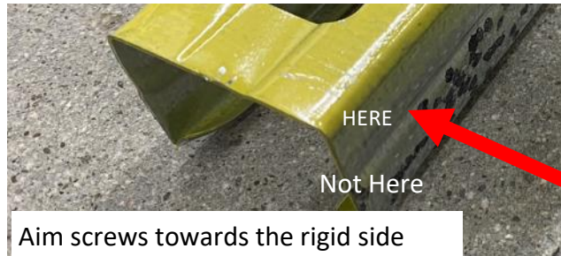
TIP: How To Screw into studs
